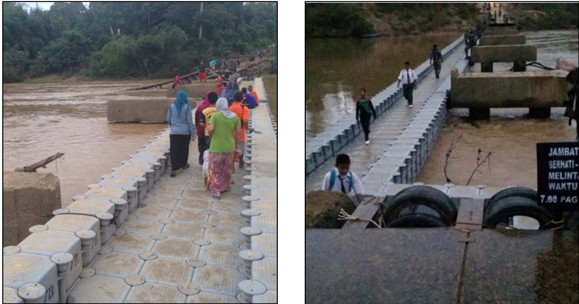
Figure 8: PFP constructed to temporary replace the collapsed bridge (Army HQ, 2016).
