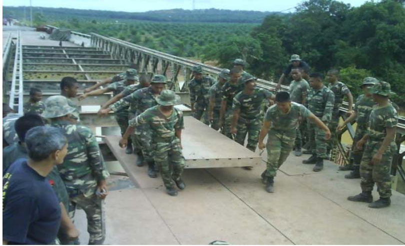
Figure 5: Compact 100 Bailey Bridge constructed during flood relief operation (Rasyid, 2008).
