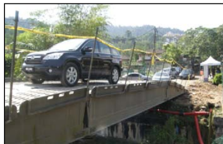
Figure 1: BR90 GSB deployed during Bukit Antarabangsa landslide (Jusoh, 2008).
