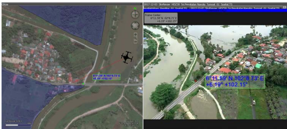
Figure 6: Location of congestion / bottleneck of flood water outflows in the hotspot area.
