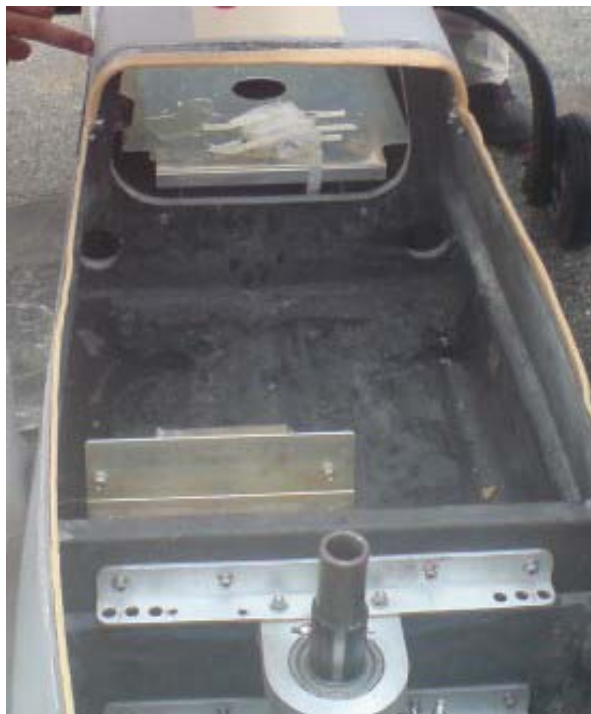
Figure 4: Water leakage found inside the fuselage
