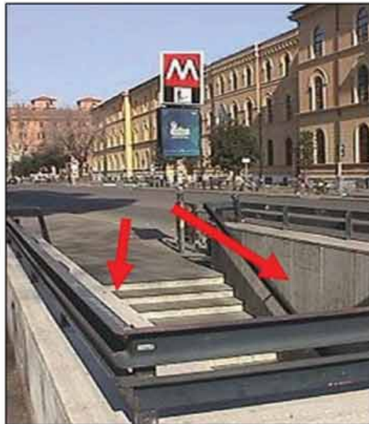
Figure 4: Positioning of the detection system.
