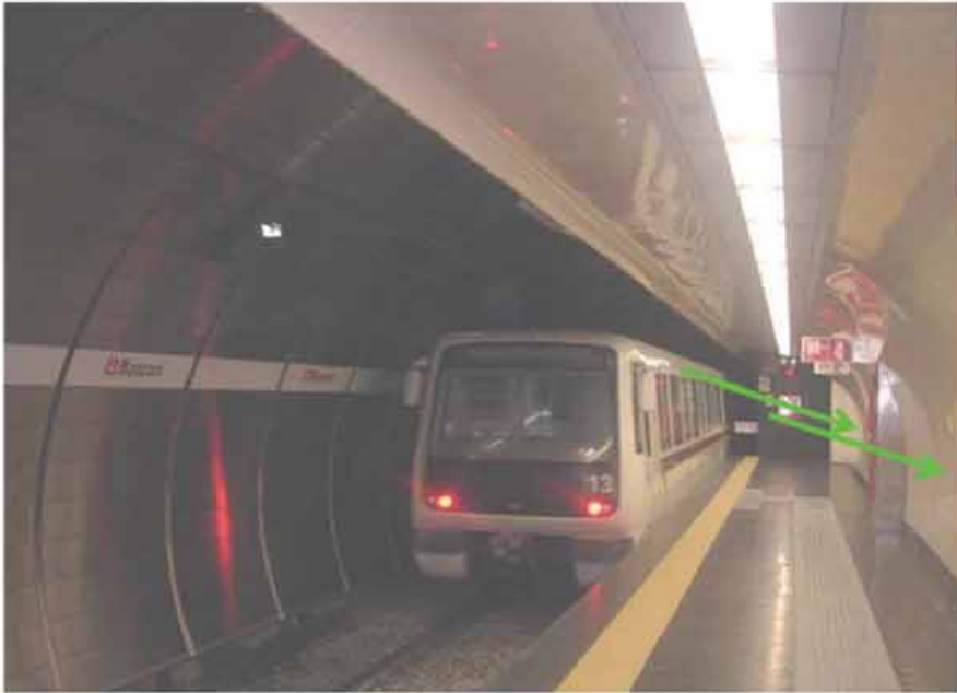
Figure 7: Positioning of the manual alarm buttons on the platform.
