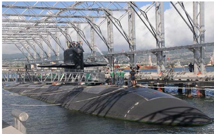
Figure 8: A Drive-In magnetic silencing facility at Kings Bay, Georgia, USA (SSFM International, 2019).
