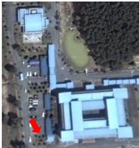
Figure 3: Test area located at N 2° 58.056' E 101° 48.586' (Source: Screen capture from Google Earth)
